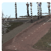
Bikepath Digital Inspection
